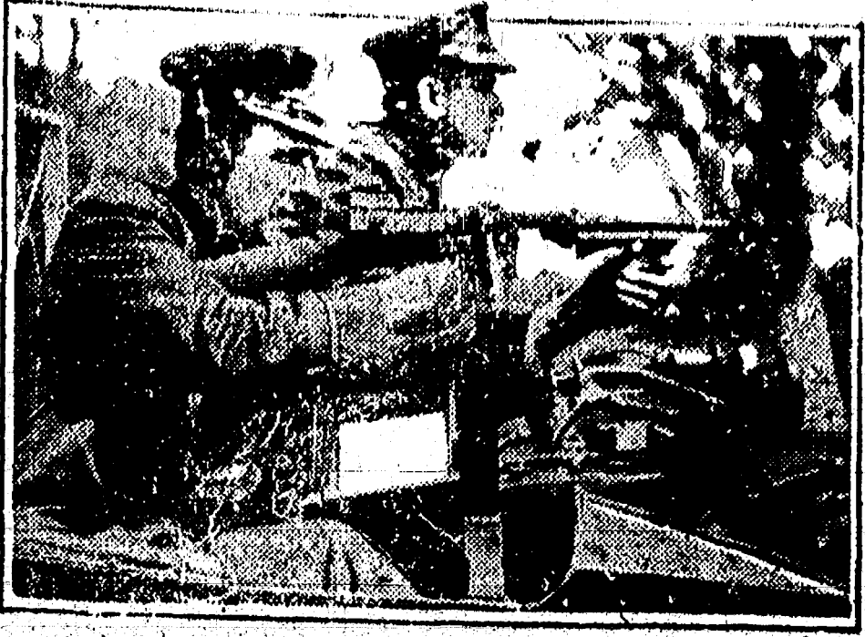
This machine gun, weighs only 9 1/2 pounds. It will shoot single balls or shot, or will fire in bursts at the rate of 1000 shots a minute. It will demolish an automobile in a few seconds. This new weapon of death is the invention of Gen. John T. Thompson, Director of Armaments during the war.
